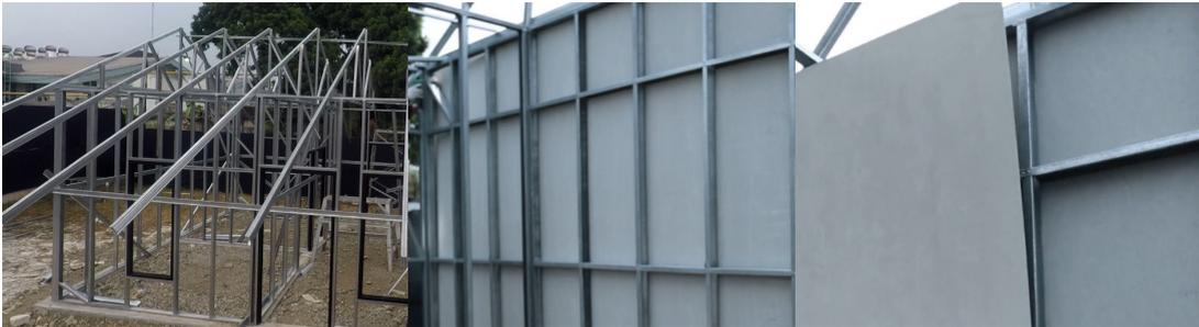
GRC Modular House - Double Wall Is a prefabricated house that uses GRC board 10 mm (outer side) and 8 mm (inner side) thick cement board that are bound by steel frames that give the walls tremendous support. The density of GRC board strengthens the building, yet still lightweight & versatile that allows for easy transport and distribution. GRC board Modular House is expected to become an earthquake-friendly building.
